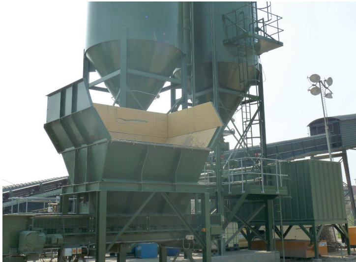
HBM Plant - Greenwich
